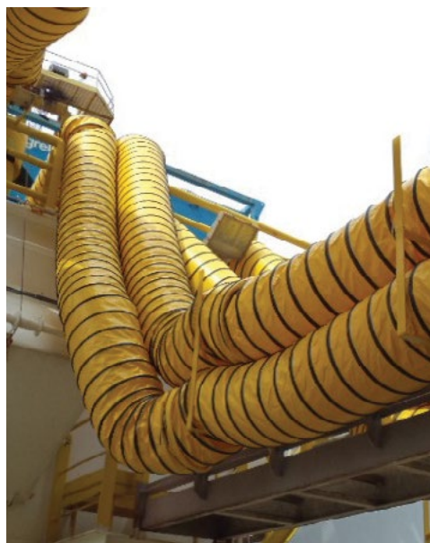
In the stacking process, ducting connects to exterior AC units and snakes through interior doors to keep the rig's interior dehumidified.
